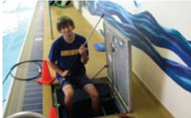
Phil Cleaning the Surge Tank
